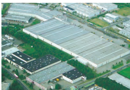
Logistic Center (approx. 60.000 m 2 )
